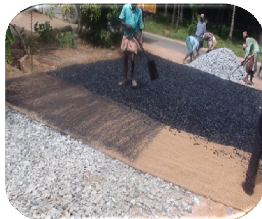
Coir Geo-textiles @Road construction
